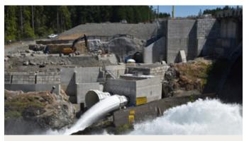
The water intake structure and low level outlet valves on the downstream side of the John Hart Dam. The intake goes under the dam with water passing into the power tunnel for power generation or to the two low level outlet valves.
